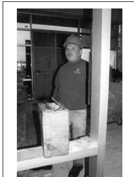
Figure 3. A subcontractor from Lurie Glass installing windows
